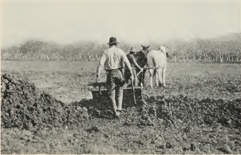
Fig. 13.—Backfilling a tile trench with slip scraper.
